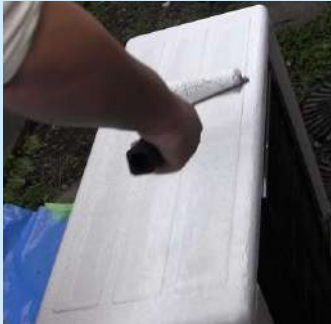
Painting Outdoor Unit Cover Coat
